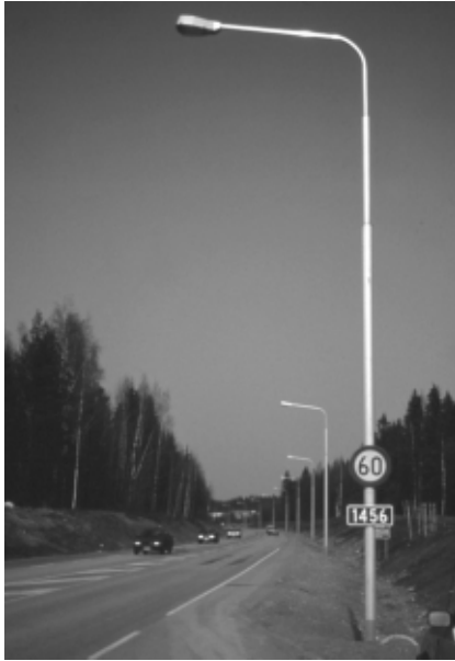
Fig. 33 Aluminum light poles are widely used around the world for their corrosion resistance, and their breakaway-base crash protection systems that provide safety for car drivers and passengers.
