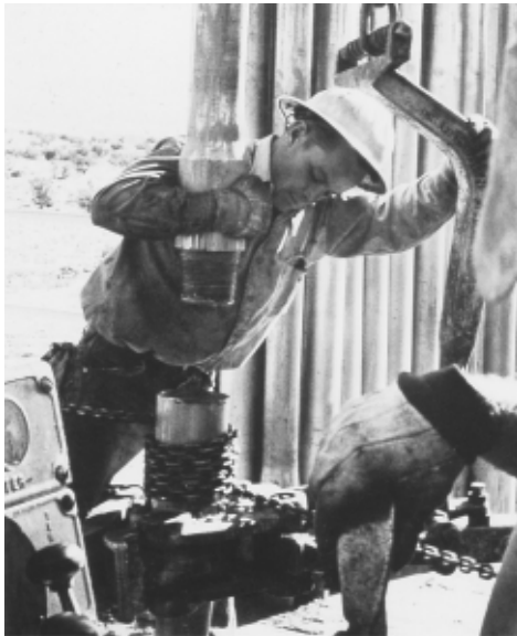
Fig. 38 Long-length drill pipe often is made of 7xxx (as well as 2xxx) aluminum alloy extruded tube.
