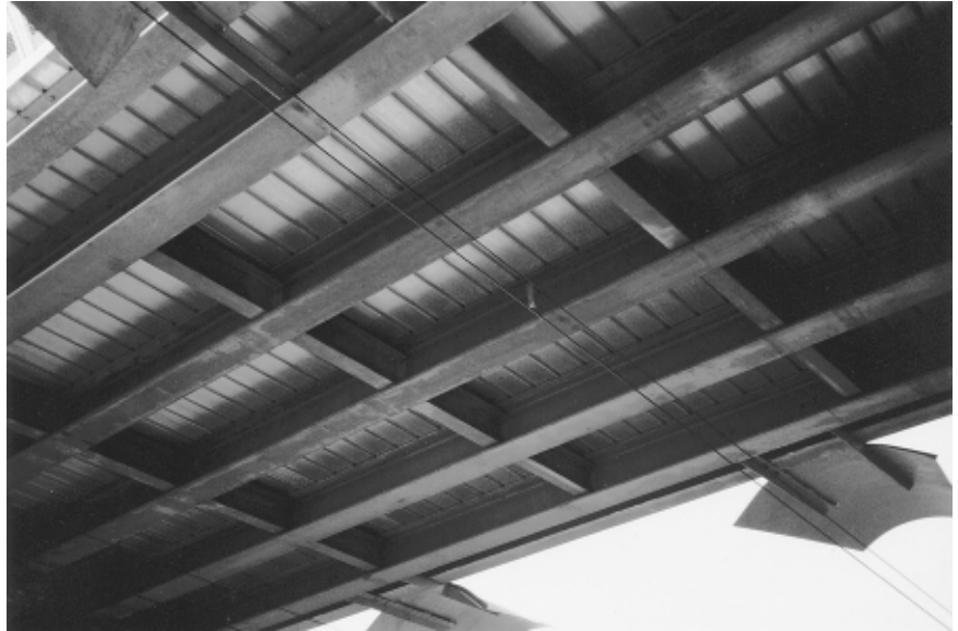
Fig. 31 Replacement bridge decks, usually produced in 6063, are readily put into the roadway in hours.
