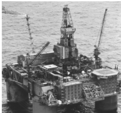
Fig. 21 The demands of the superstructures of offshore oil rigs in high humidity and water exposure are met with 5454, 5086, and 5083 aluminum-magnesium alloy welded construction.
