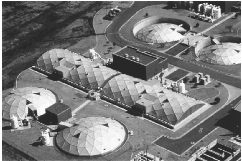
Fig. 25 Sheet of 5xxx alloys often forms the surface of geodesic dome structures, as in this example of a water treatment plant.
